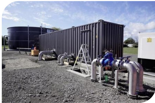
Figure 27: Hastings District Council small community water supply upgrades
