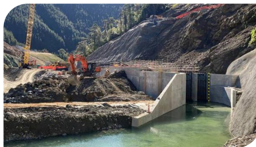
Figure 33 Waimea Community Dam currently being constructed
